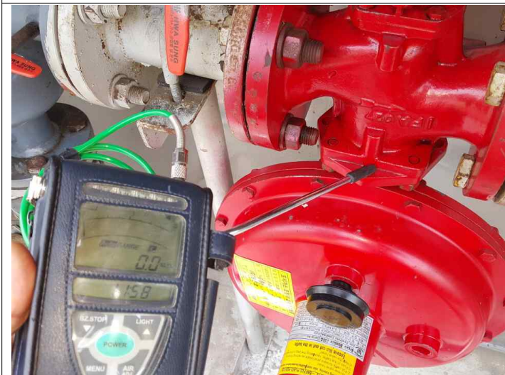
( REGULATOR 점검완료후 GAS 누설점검 )
